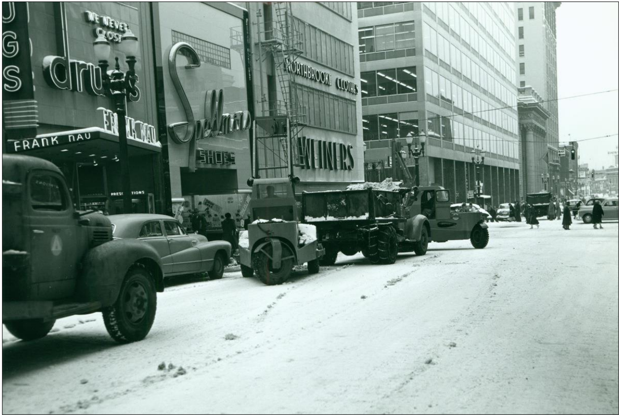
Here's a great photo from 1952 showing snow removal along SW Sixth Avenue in downtown Portland. Note the late 1940s Buick sedan up against the curb, 1947 or 1948. The two snow removing machines are locally designed "Scoopmobiles." (Source: Portland Archives and Records Center, A2001-007.576)
